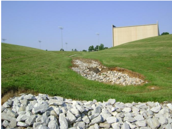
Figure 8. Mowed hill slopes adjacent to drainages east of auxiliary library facility.
