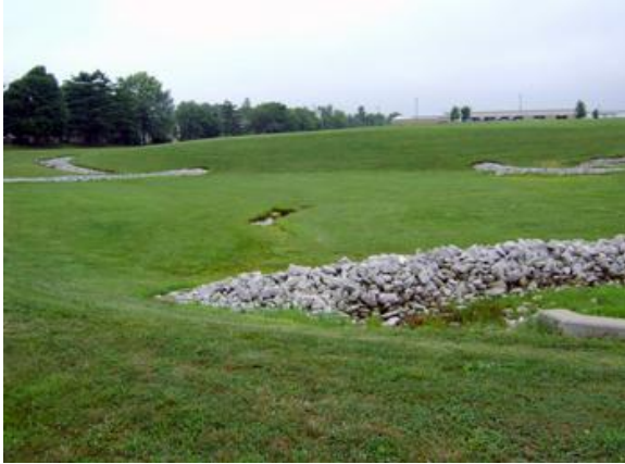
Figure 10. Confluence of three major drainages from developed area at Range Rd. and E. 14 th street.
