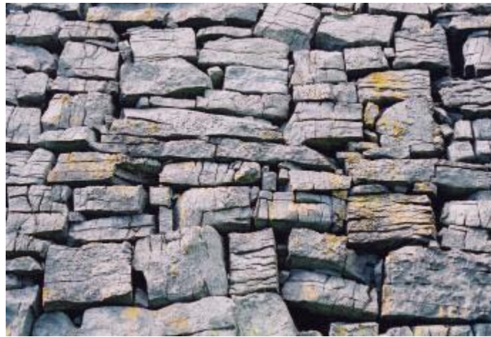
Appendix 1-2: Walls made of this stacking limestone are seen along 3 rd Street as well as throughout campus.
