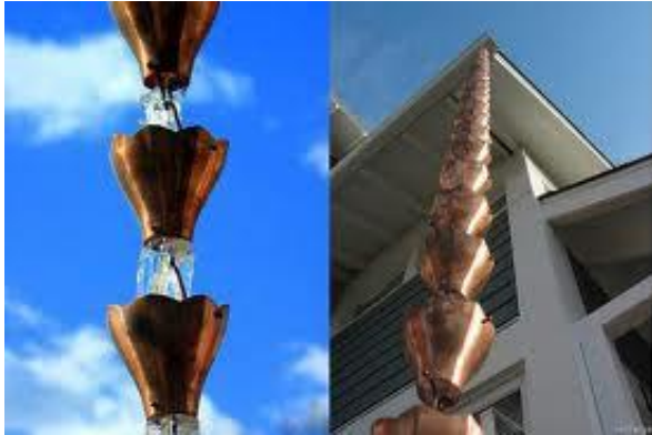
Japanese Rain Chain- downspout alternative ( http://greenupgrader.com/tag/rainwater-harvesting/ )
