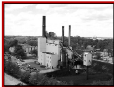
Central Heating Plant #5 Circa 2000
