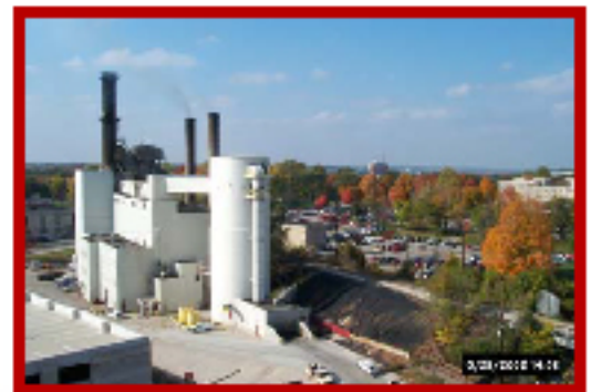
Central Heating Plant #5 Circa 2003
