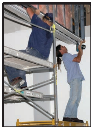
Tim Hobson and Mike Baker of the carpentry shop.
