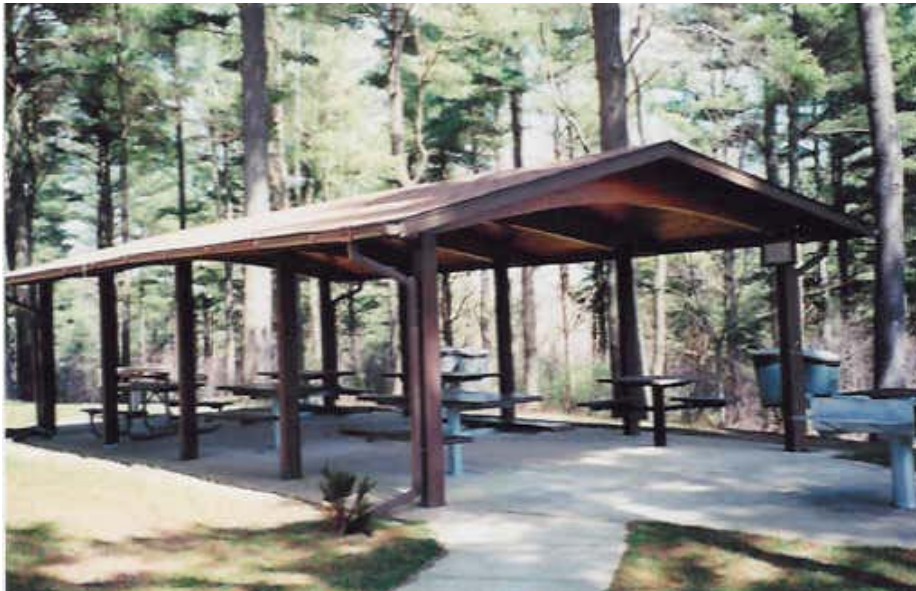
Picnic shelter at Barre Falls Dam, Hubbardston, MA. Photo courtesy of the U.S. Army Corps of Engineers.
