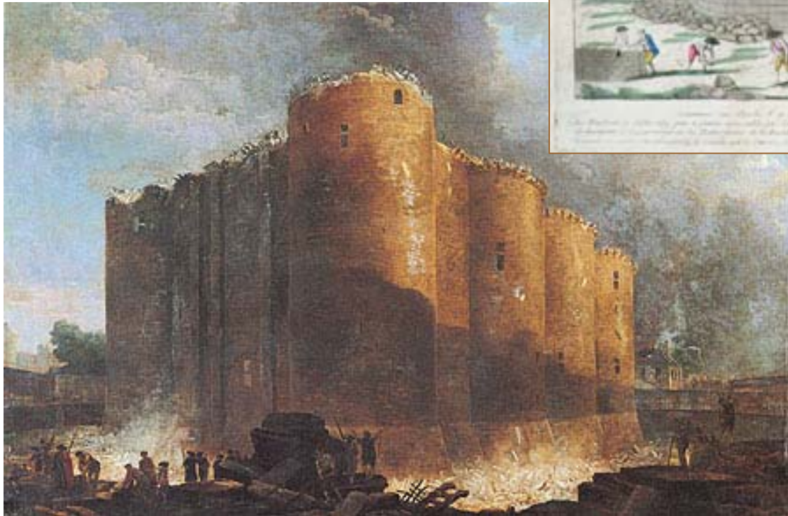
The Bastille in its first days of demolition, Robert Hubert, 1789
